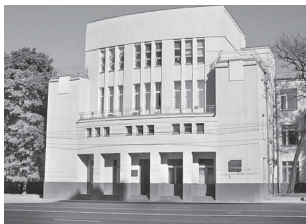
Fig. 1. G. M. Krzyzanovsky Moscow Power Engineering Institute (19 Leninsky Prospekt). The building was constructed for the Biomedical Institute at the Directorate of Scientific, Artistic and Museum Institutions for the Russian Soviet Federated Socialist Republic.
